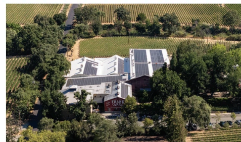
In 2024, the winery installed 800 solar panels atop its facility.
