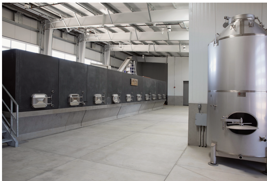
Zialena Winery ferments all red wines exclusively in cement tanks by Sonoma Cast Stone.
