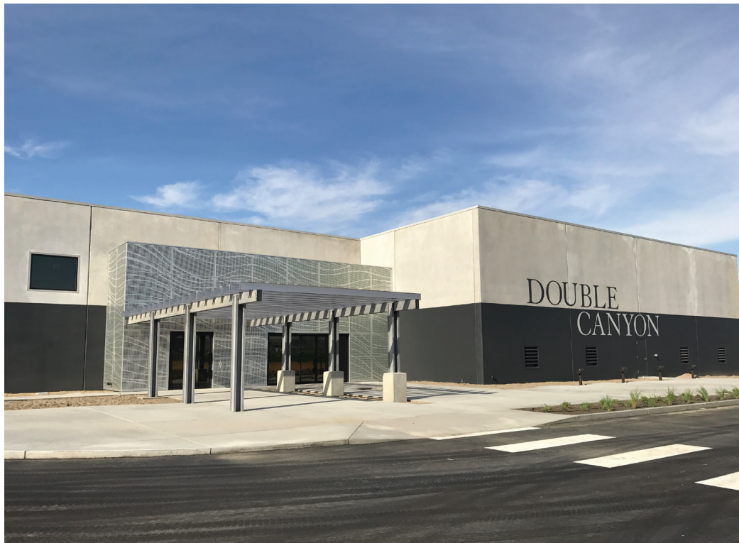
Double Canyon’s tilt-up walls are insulated to protect it against the temperature extremes of the Washington desert.
